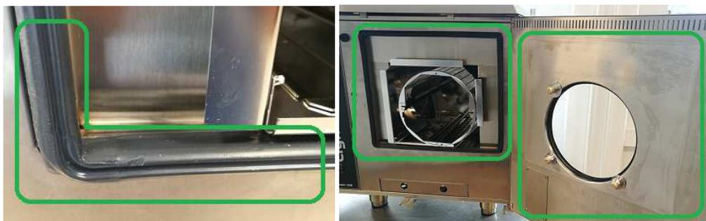
Figure 27 – Clean any residues in the door seal gasket as well as the door panel.
